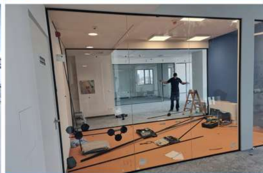
COMMERCIAL FACILITIES - Sirius, glass partitions
